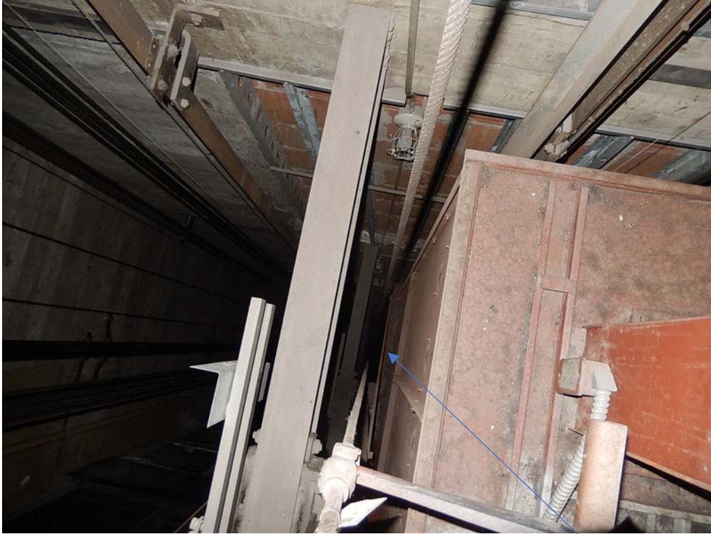
The platform can be seen in its typical rectangular shape here.
